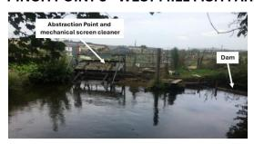
West Mill Fish Farm abstraction point, mechanical screen cleaner and dam. In certain flows, smolts get trapped and are killed by the mechanical screen or are subject to predation. The dam has been removed (January 2025) but could be reinstated in the future
