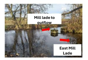
Before the main lade outflow there is a split in the lade which allows water down the old East Mill Fish farm abstraction point. Smolts could easily be diverted down this East Mill exit and probably get lost because it is has significant barriers over its length before its outfall into the river.
