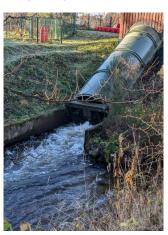
The Hydro turbine – an Archimedes screw system which allows smolts to enter and journey through the screw – although classified as "fish friendly", damage to some smolts is likely, leading to death.
